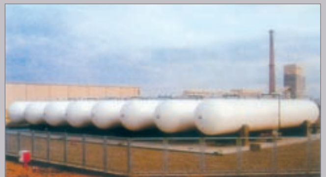
Eight 207 m 3 tanks at a glass factory
